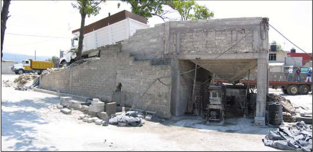
Figure 3. A Two-Story Block Production Facility ( Blockera Sobre Desnive ).
